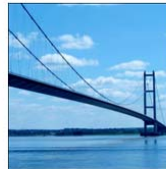
The Humber Bridge
